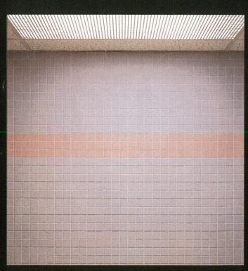
The photographs above illustrate the dramatic difference the placement of overhead lighting can make in the appearance of a tiled wall. The photographs on the left show the effect of overhead lighting panels mounted next to the wall resulting in "wall wash." This harsh lighting technique creates harsh shadows that accentuate any irregularities in the tiled surface.
